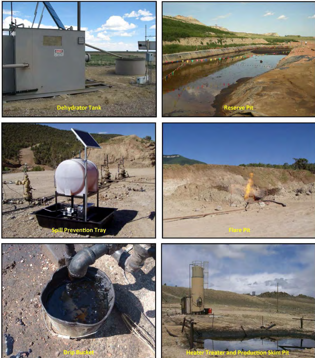
Figure 1. Hazards to birds in oil and gas production facilities.
